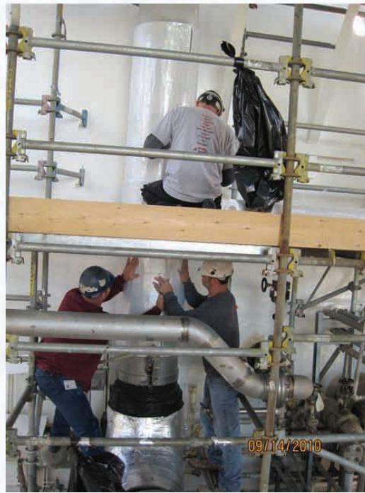
TOP: Vapor stop applied above the clamp band CLOCKWISE FROM LEFT: Clamp band applied over the Cryogel®; Failed urethane insulation; Insulators working on different levels; Cryogel® insulation being applied
