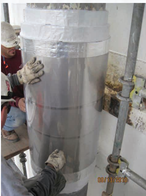
TOP: Vapor stop applied above the clamp band CLOCKWISE FROM LEFT: Clamp band applied over the Cryogel®; Failed urethane insulation; Insulators working on different levels; Cryogel® insulation being applied
